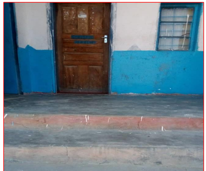
Figure 9: Classroom building with door steps
